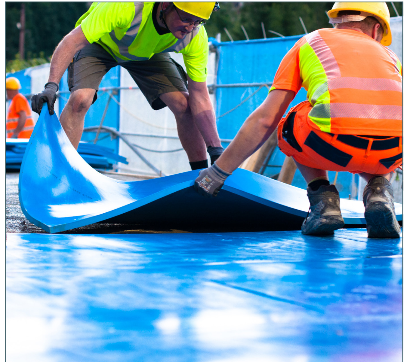
Installation of PURASYS MSS to provide elastic support in the track bed
